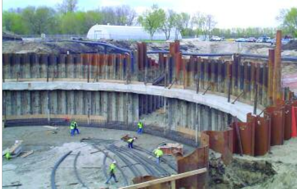
Sheet pile wall installation using reinforced concrete rings for lateral support.
