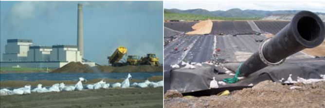
Ash landfill construction.
