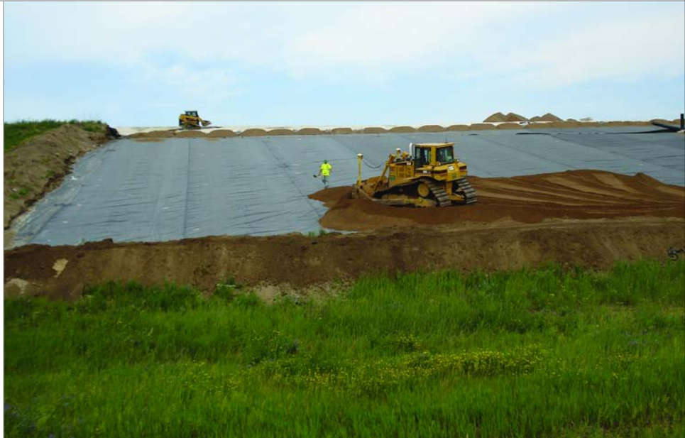
Placement of geotextile liner.
