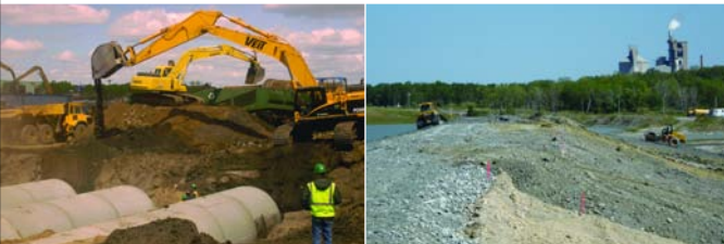
Installation of storm water control system.
