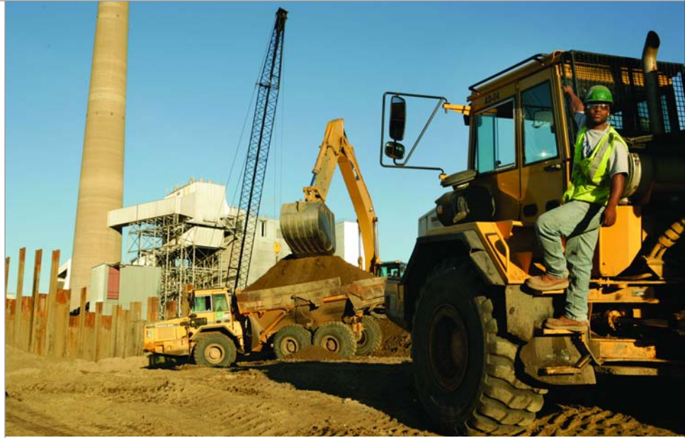
Mass grading, excavation, and sheet pile installation.
