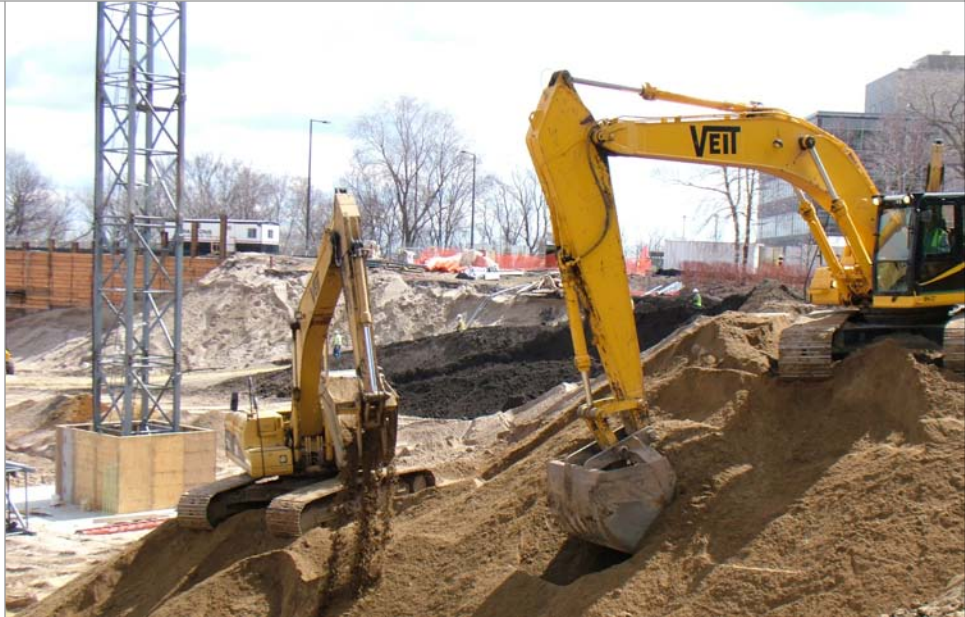
Mass excavation for multistory office tower.
