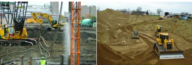
Excavation and piling installation for University of Minnesota football stadium.
