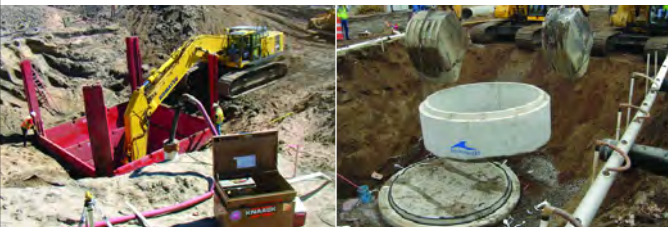
Sanitary sewer lift station installation.
