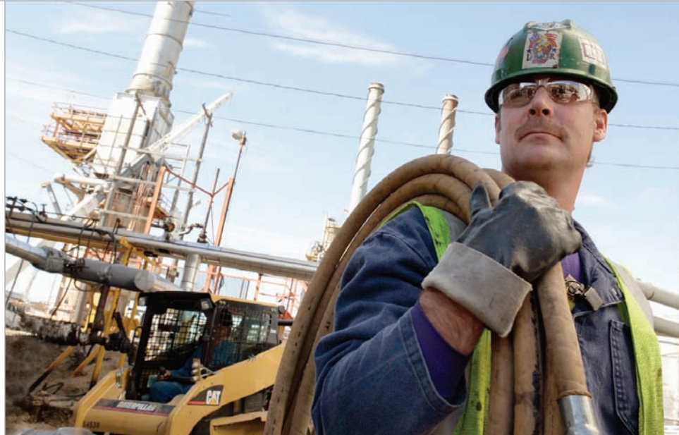
Veit workers tackle cleaning at a petroleum refinery.
