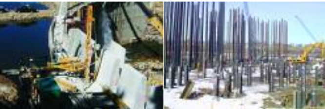
Strand anchor placement, Tarryall Dam, Colorado.
